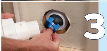
Take disposable cutter out of the evacuation fitment and turn the cutter around so teeth are facing the membrane. Gently reinsert the cutter into the 2" evacuation fitment.
