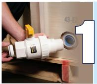
Remove the 2" screw cap from the bottom 2" flange of the bag liner. Screw this same 2" cap into the outbound side of the food grade valve.
